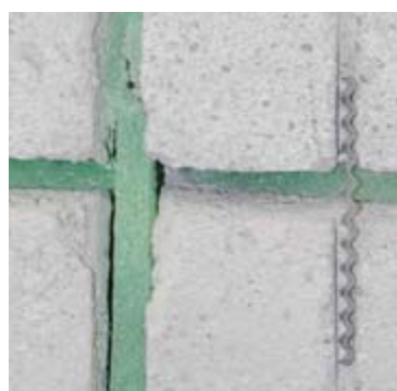
Joint with filler material
