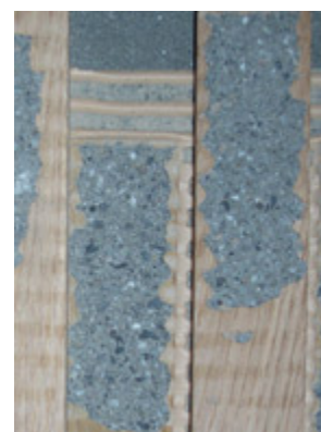
Cohesive failure in substrate
