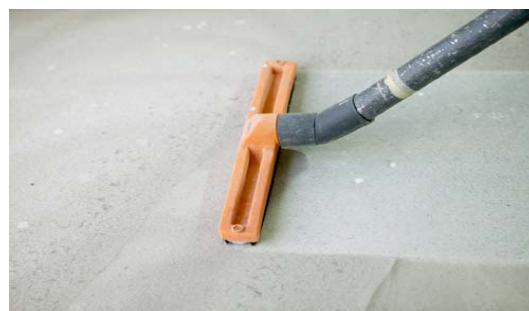
Removing dust with an industrial vacuum
