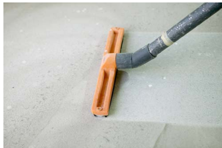
Removing dust with an industrial vacuum.
