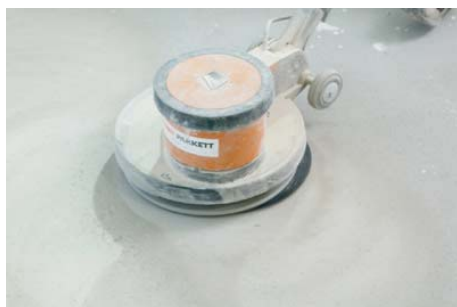
Full surface grinding.
